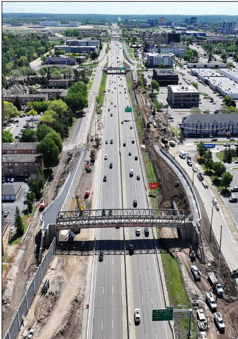
Work is underway on a major state and federally funded project to improve I-494 from TH 169 to the MSP Airport. The first phase, scheduled to be completed at the end of 2026, includes significant improvements to I-494/I-35W interchange, several new bridges over I-494, and a new E-ZPass lane between East Bush Lake Road and I-35W.
