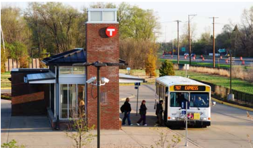
The 494 Corridor Commission has successfully shifted 2,238 “drive alone” commuters to alternative modes, thereby reducing congestion in the 494 corridor.
